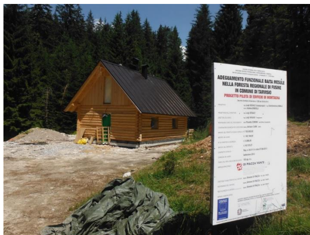
Figura 6 - Baita Mesule - work in progress
